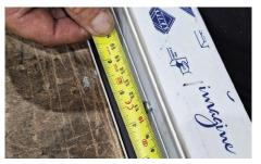
Measure the position of the glazing clip fixings
