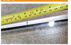
Mark them on the window previously removed, do not forget there is a gap of approx. 8mm around the glass.
