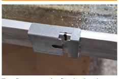
The clips can now be fitted to the glass DGU (double glazed Unit) Top and sides only. The top clips will slide towards the outside of the window frame when securing the DGU. The side clips will slide down the frame when securing the DGU.
