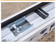
Put the bottom clips on the frame, slide in and then towards the outside of the window and place the packers into position.
