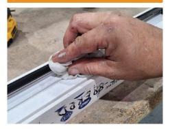
Clean the rubber seal around the window frame to remove any possible grit or grease.
