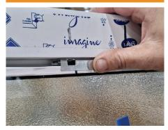
Line up the glazing clips with the screw in the frame, and slide into place.
