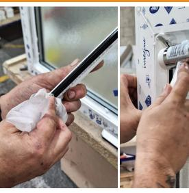
Starting with the shortest bead, wipe the rubber seal and tap the beads into place.
