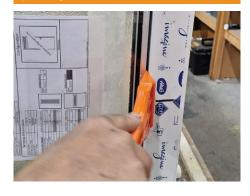
Adjust the position of the DGU to centralise and leaving an equal gap all the way around.
