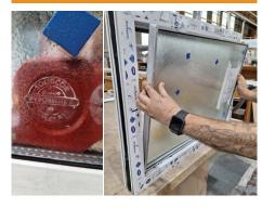
Check the window is the correct way around, so the fire glass is on the inside and lift into place. Pyrobelite is the Fire Glass and is clear
