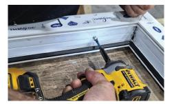
Inside the frame you will find some pre-drilled holes. Insert the dome head screws provided, leaving them approx. 2mm away from the frame so that the clips will slide on later.
